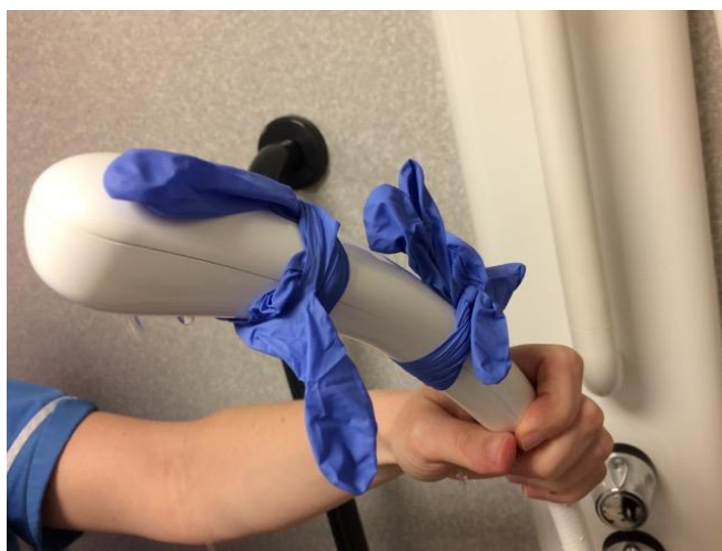
The damaged Medi-Shower outlet repaired by ward staff.
